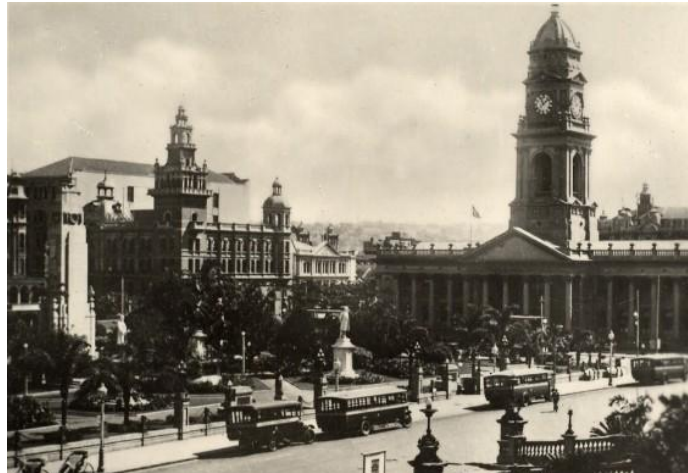
Durban Inner City Central Post Office (historic). SOURCE: EThekweni Municipality Archives, 2021
